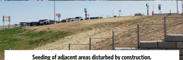
Seeding of adjacent areas disturbed by construction.
