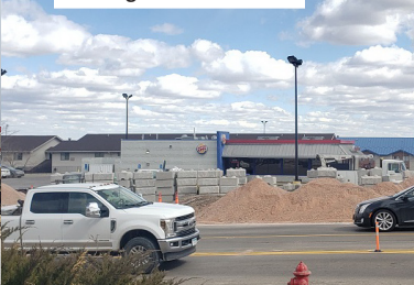
Retaining Wall Construction
